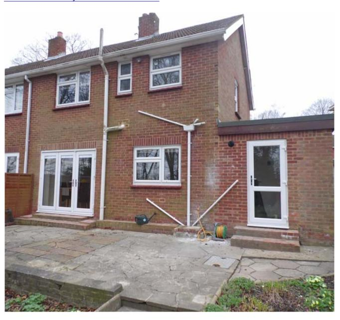
As part of the extensive renovations at this property, new uPVC windows and doors were installed to both improve the aesthetics and reduce the heat loss potential of the property.
